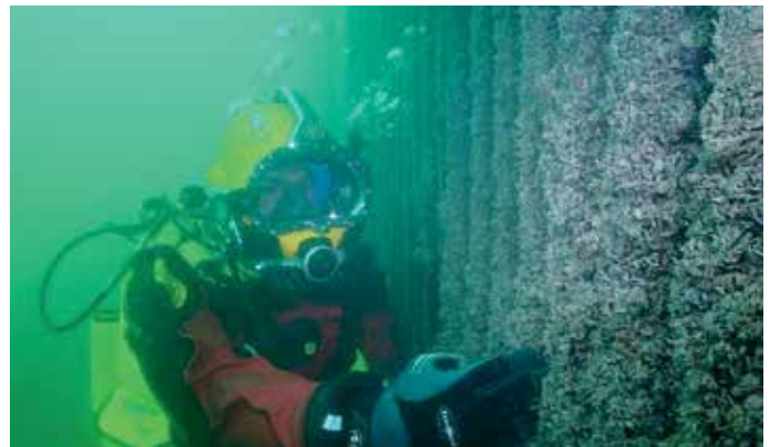
Removing quagga mussels from trash racks at Whitsett Intake
