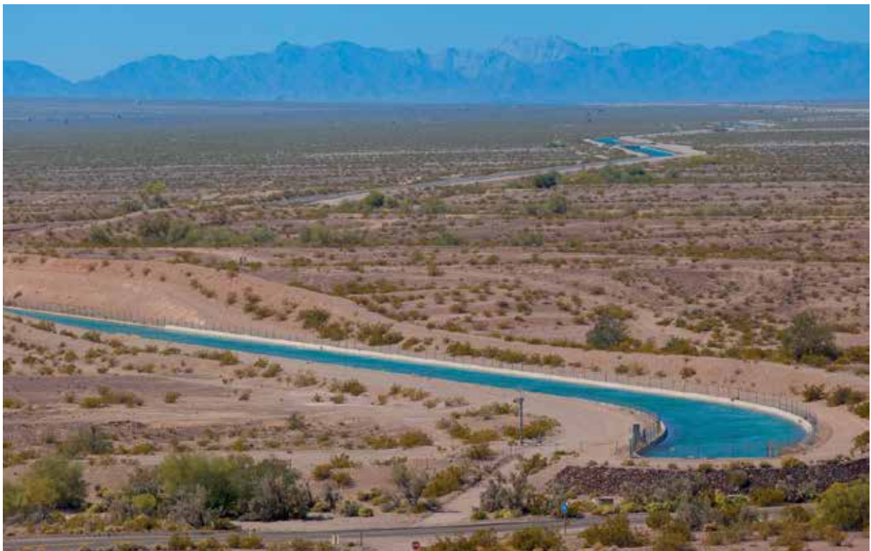
Colorado River Aqueduct
