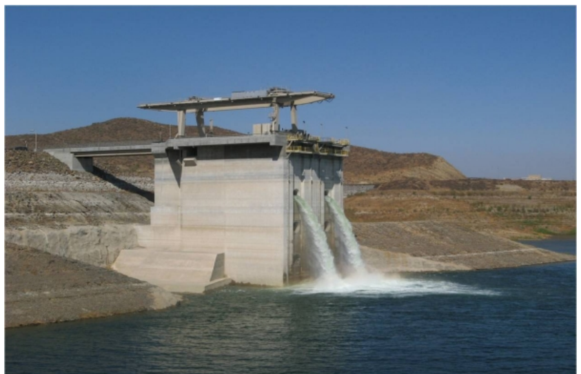
DVL Inlet/Outlet Tower during filling operations.
