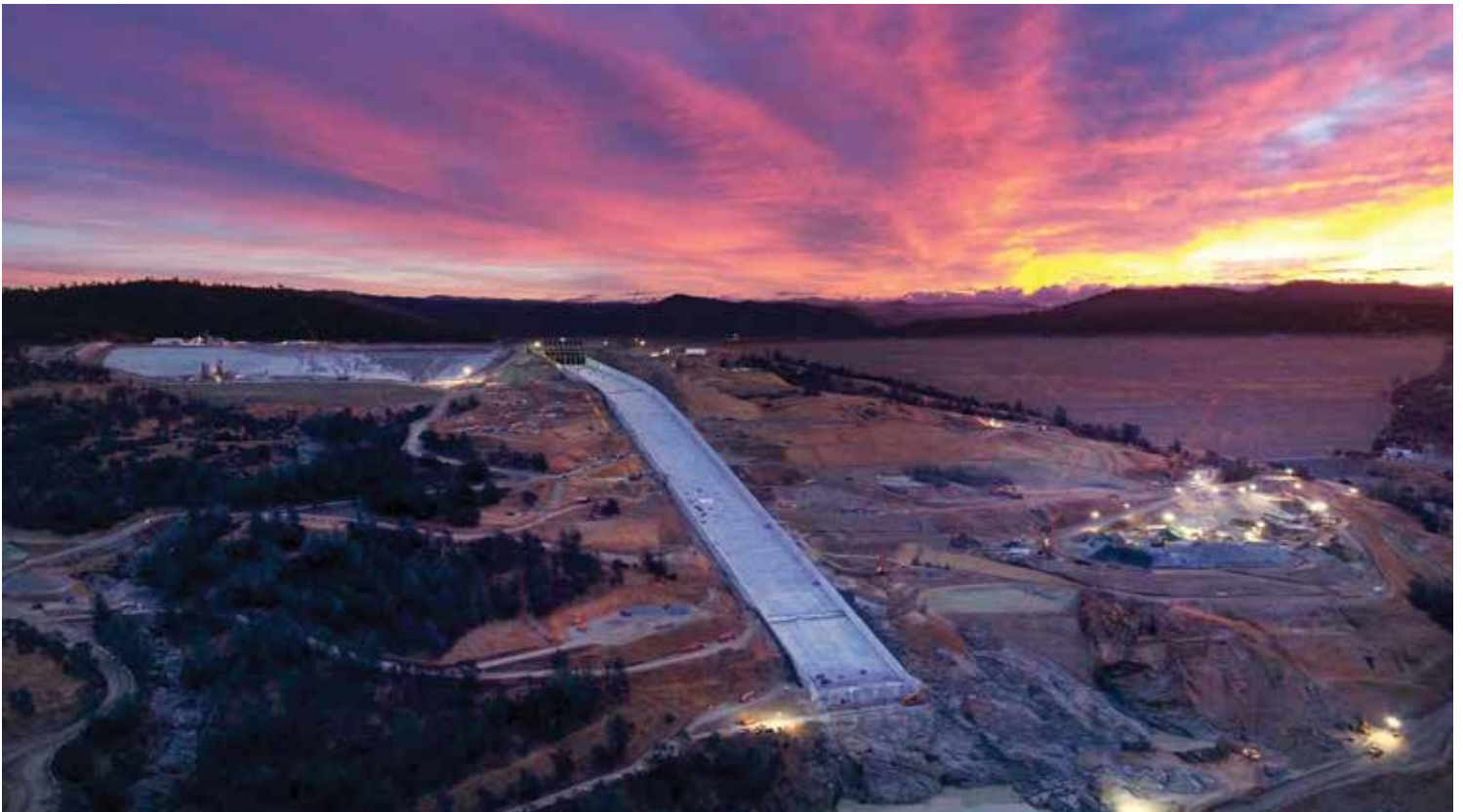
Lake Oroville main spillway, October 2018 Photo courtesy of DWR
