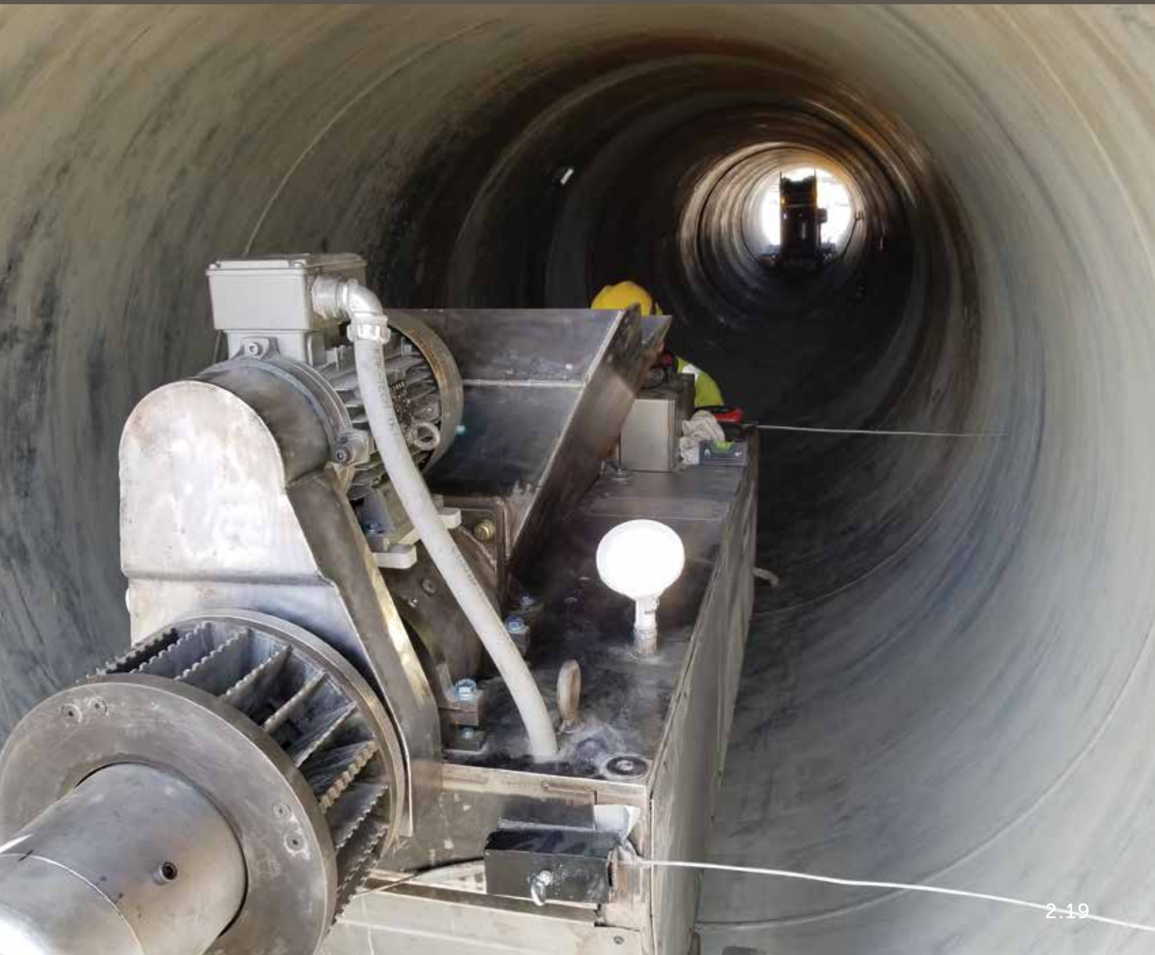
Cement mortar lining machine on the Second Lower Feeder
