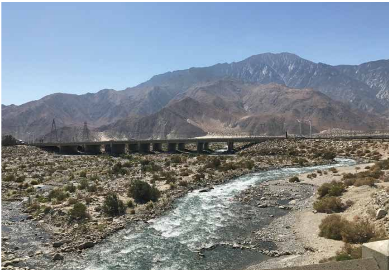
Deliveries at Whitewater River near the 10 Freeway
