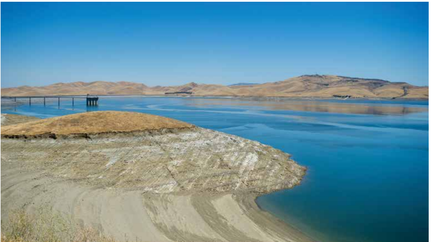
San Luis Reservoir, July 2018 Photo courtesy of DWR
