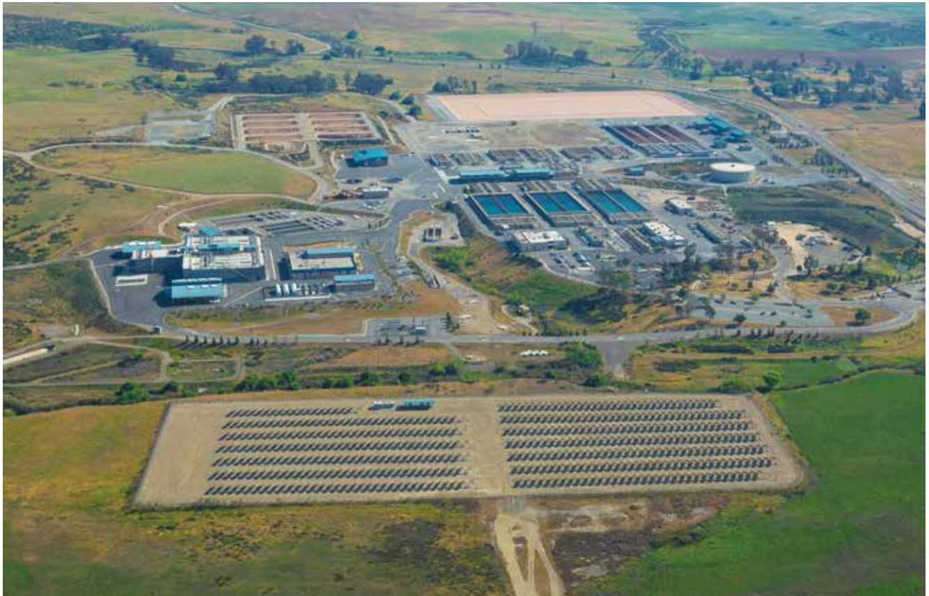
Aerial view of Robert A. Skinner Water Treatment Plant and solar farm
