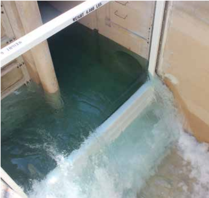
New weir gate near DWCV connection
