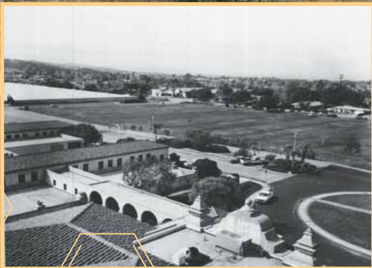
PICTURED LEFT, A VIEW OF THE NEW LABORATORY SITE LOOKING SOUTHWESTERLY FROM THE TOP OF THE ADMINISTRATION BUILDING, 2.24.1983.
