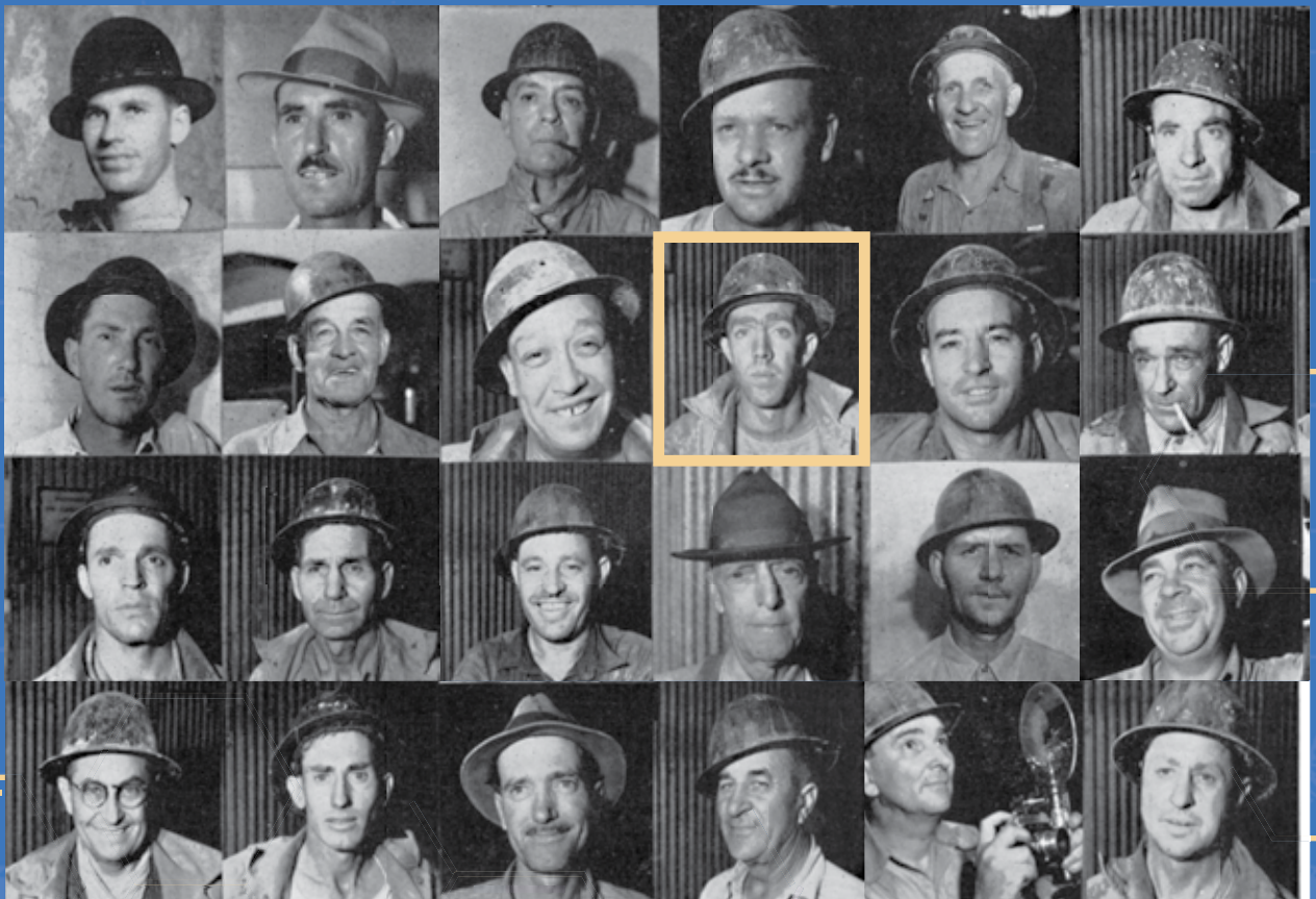
THE SAN JACINTO TUNNEL CREW, CIRCA 1939
