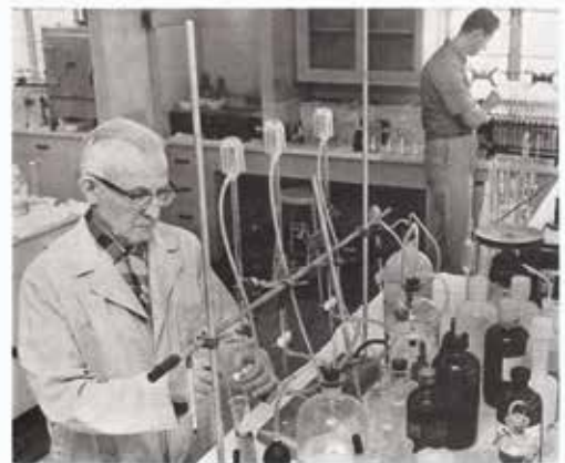
MWD CHEMIST LOUIS GIMAN RUNS WATER HARDNESS TEST IN LAB. Paul Evans, chemist, (background) checks sample for manganese content.
