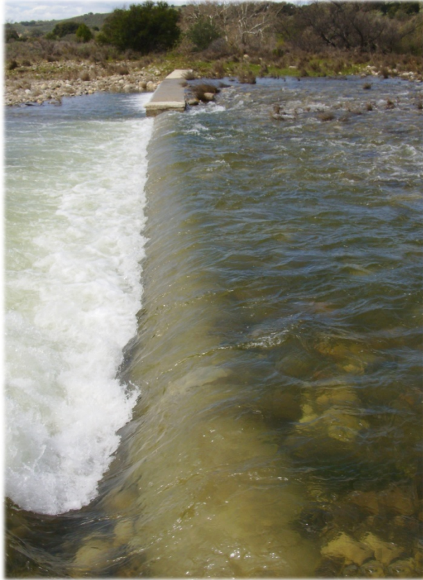
Santa Ynez River Pipeline Exposure
