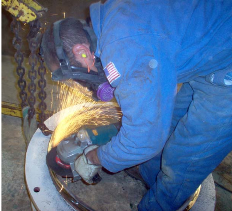
Distribution Technician Jim Thompson
