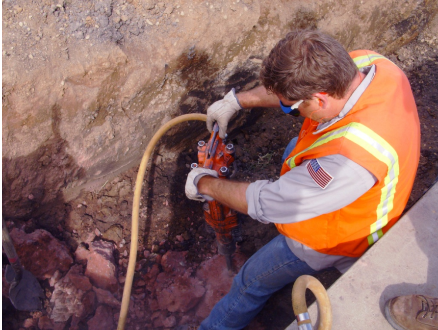
Distribution Technician Eric Kieding jack hammering at ISO#2
