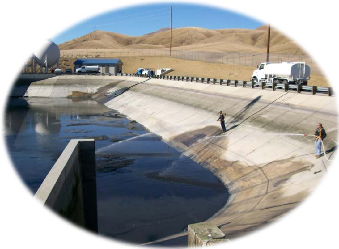
Removing Sludge from DWR Forebay
