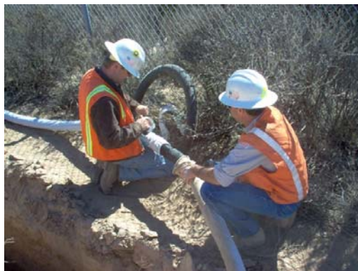
Installation of drain line
