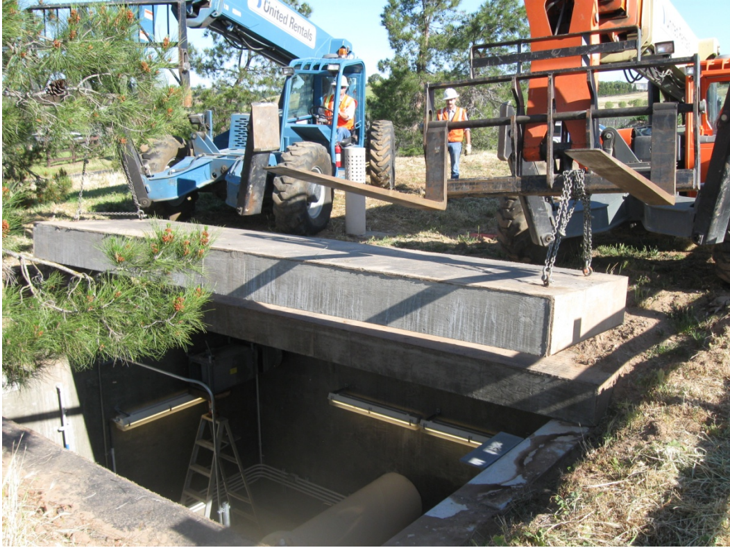
Replacing SYPS Outlet Vault Lid
