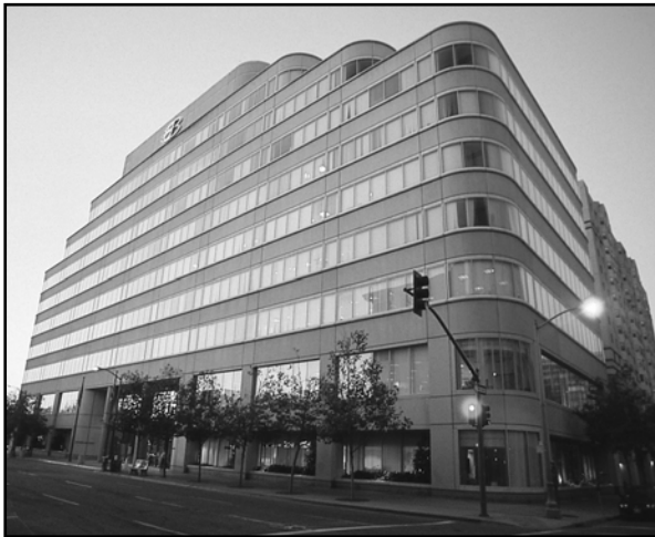
Administration Building 375 Eleventh Street, Oakland, 94607
