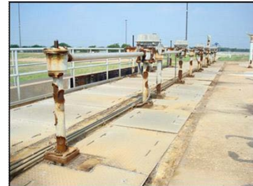
Photo 6 – Pre-aeration Tank Slide Gates
