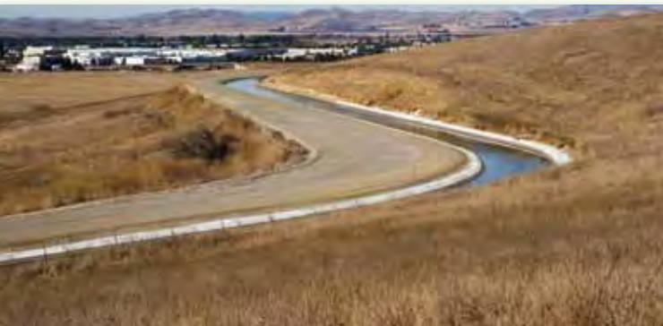
State Water Project's South Bay Aqueduct
