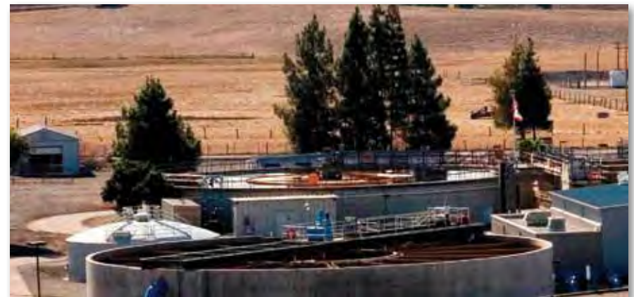
Patterson Pass Water Treatment Plant
