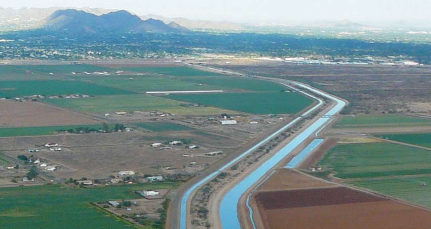
A SECTION OF THE CENTRAL ARIZONA PROJECT (CAP) NEAR TUCSON, ARIZONA.
