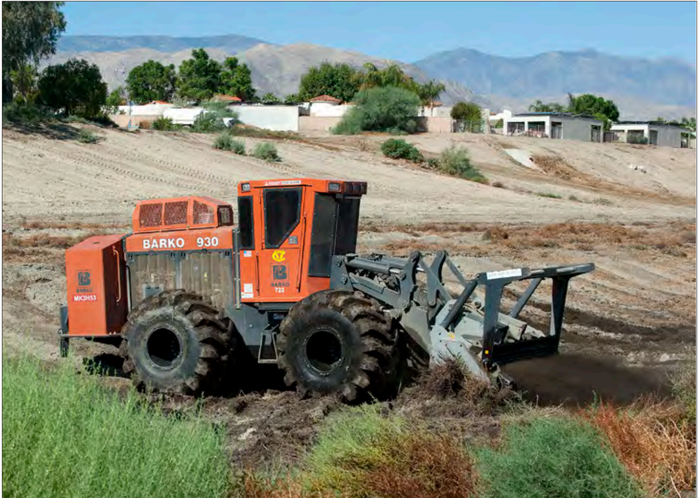
Barko mulcher clearing vegetation in the stormwater channel
