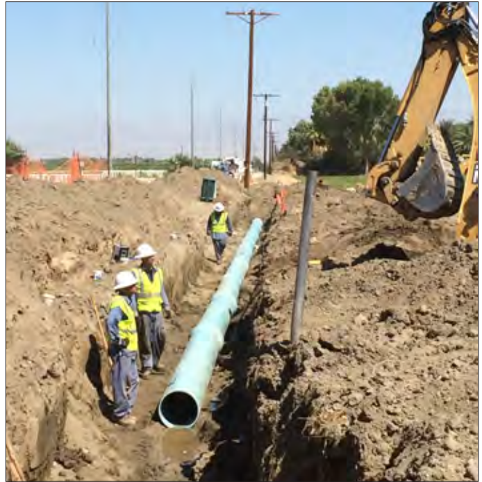
Laying Canal irrigation lateral
