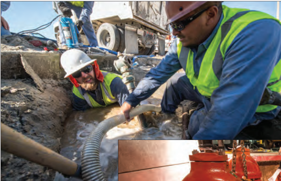
Domestic operations at work
