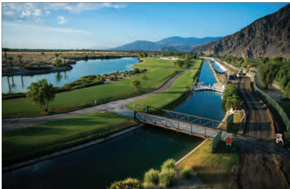
Canal relocation project at SilverRock
