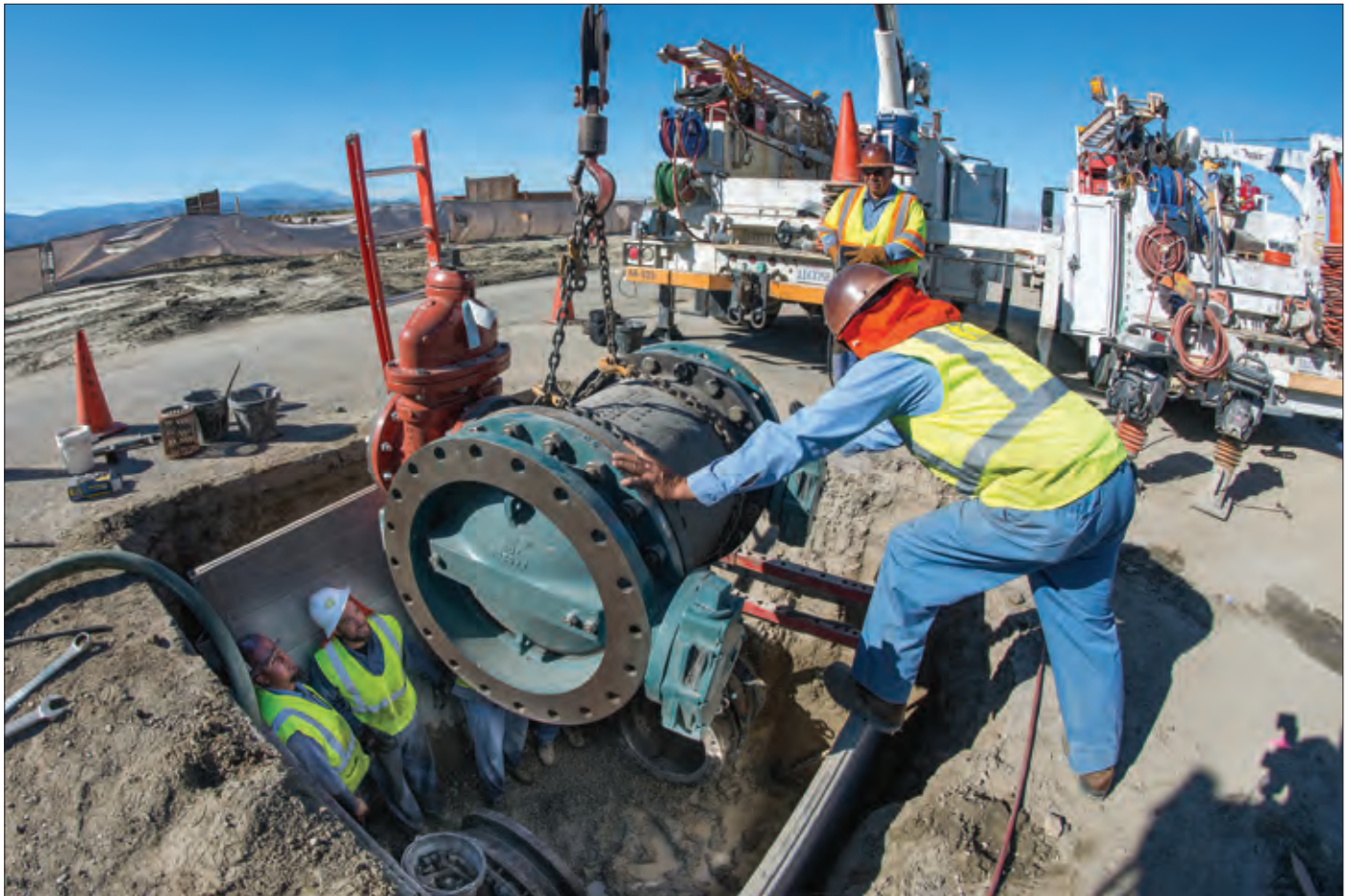
Thermal Club water main tie-in
