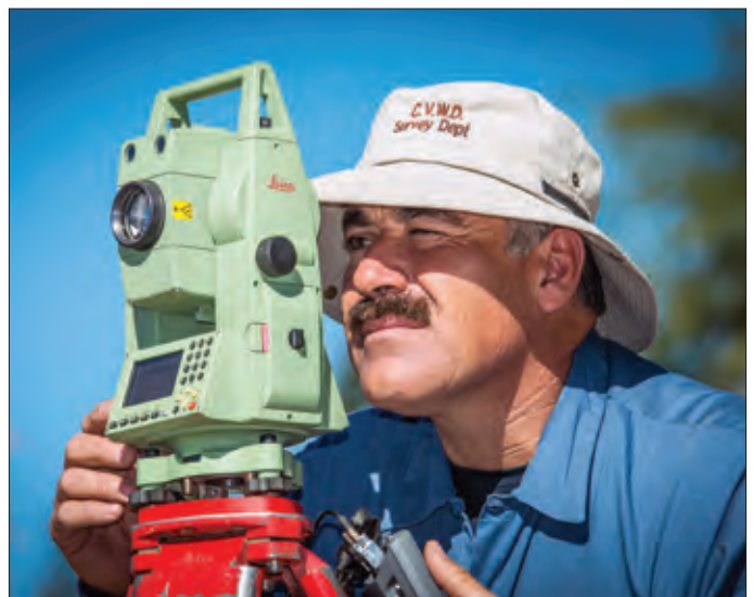
Surveying for District right-of-way
