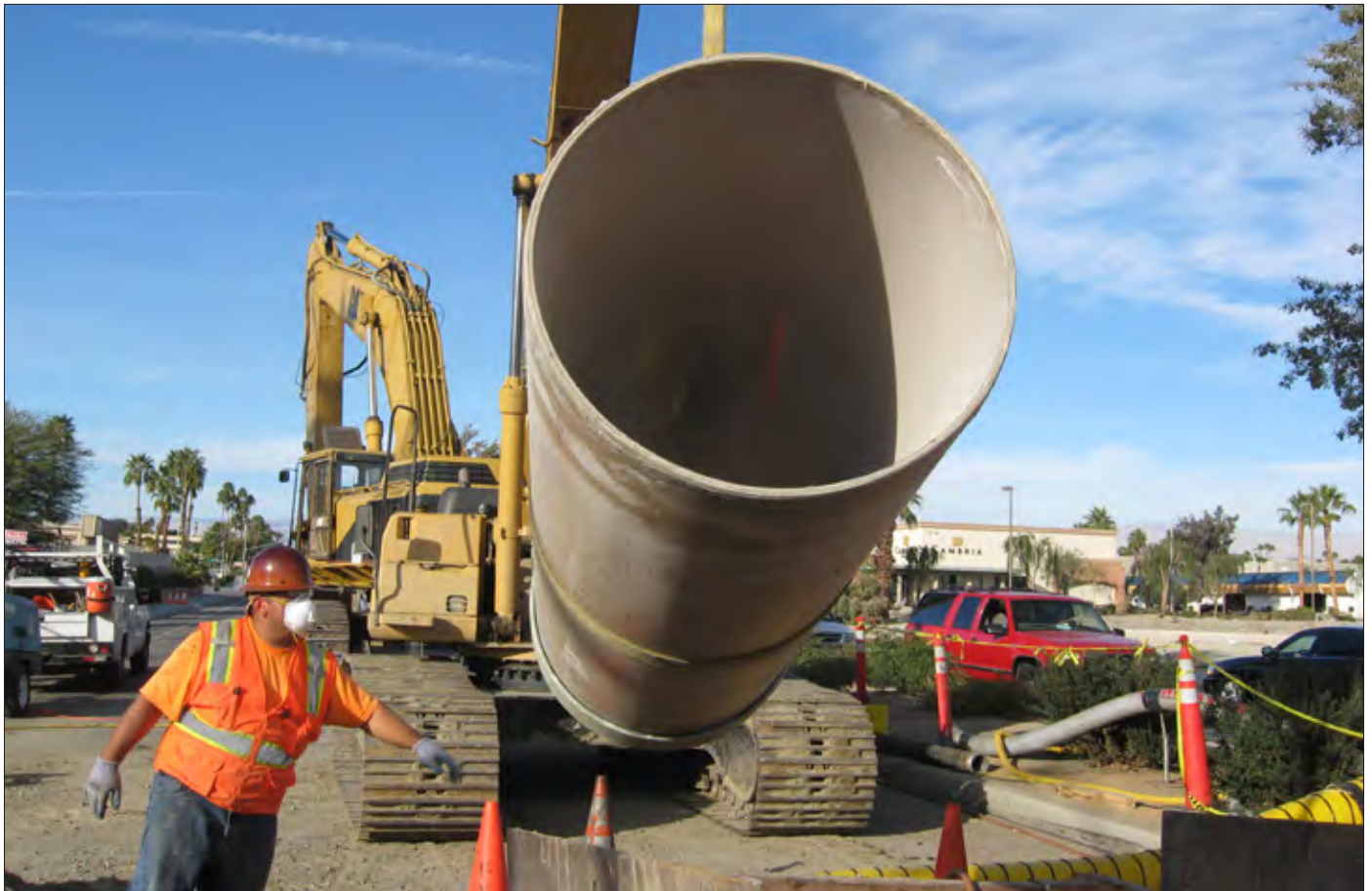
Cook Street sewer project
