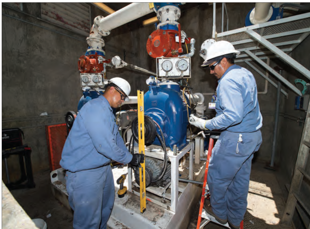
Lift station rehabilitation
