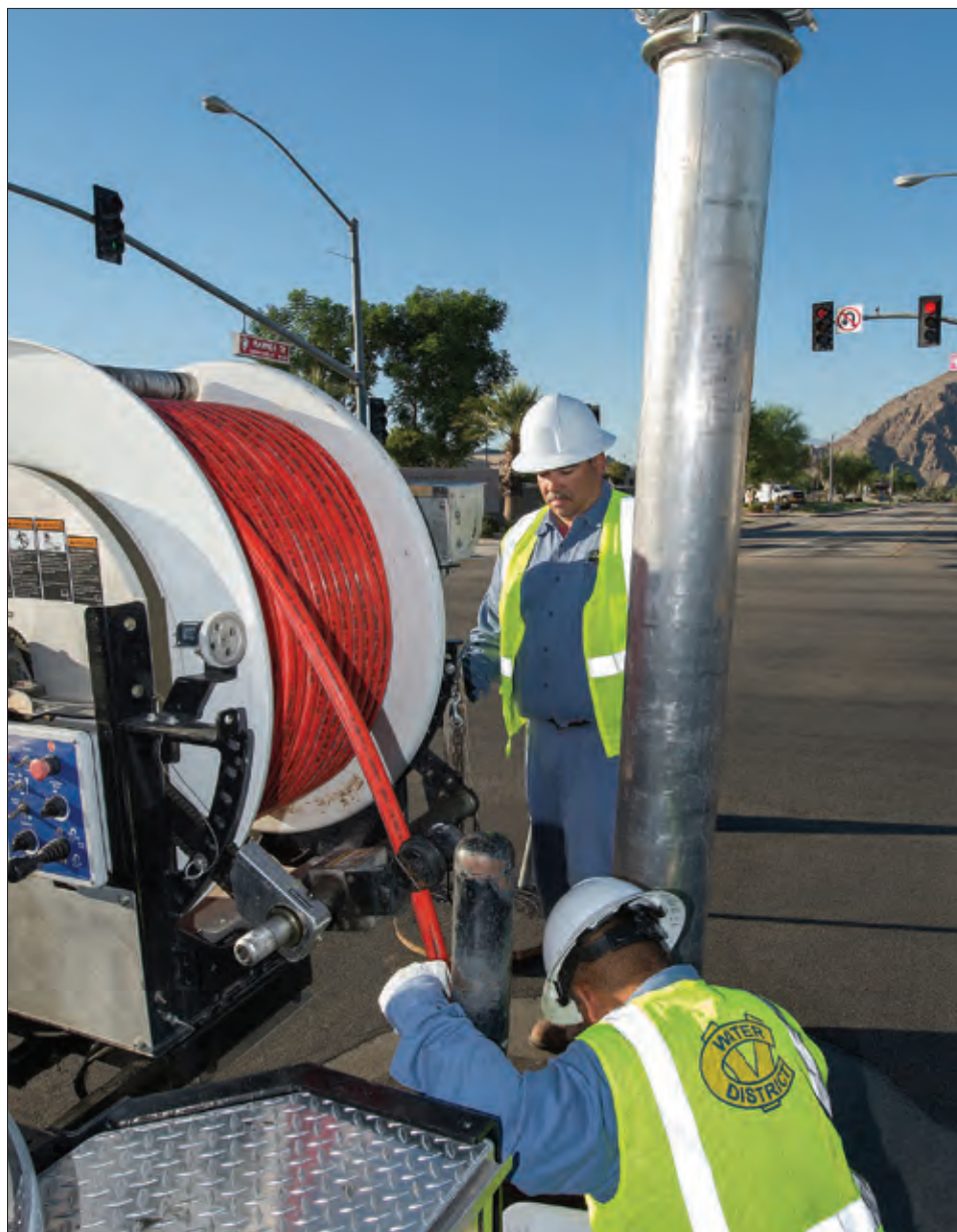
Sanitation using a vactor truck to clean a sewer line
