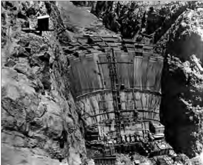
Building Hoover Dam
