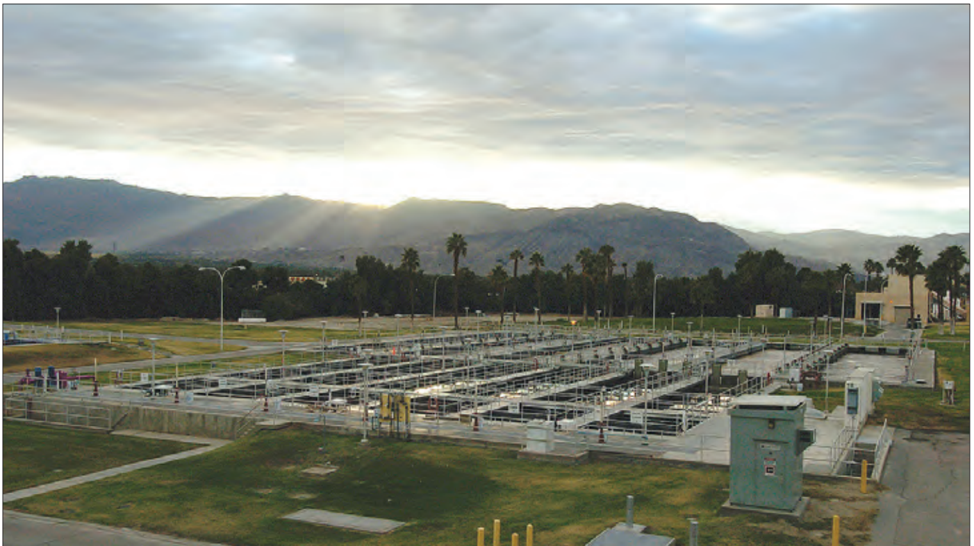
WRP 10 - the District’s largest treatment plant
