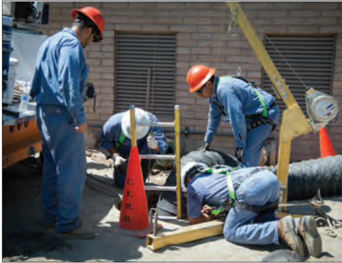
Lift station repairs
