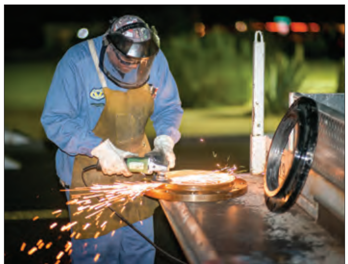
Stub out valve installation
