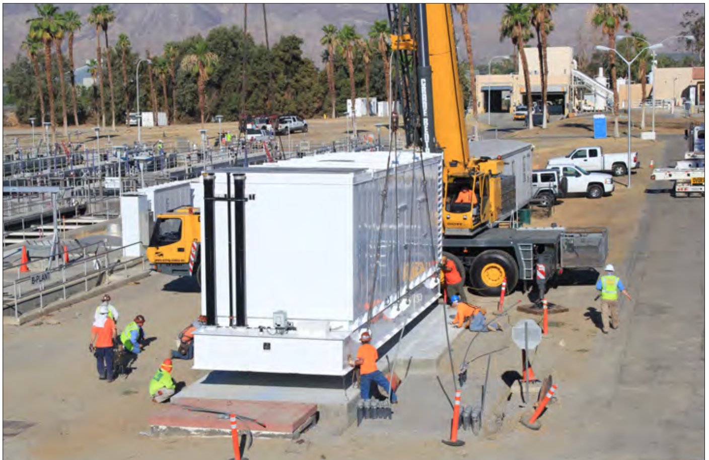
Generator installation at WRP 10 - Air Process Improvement project
