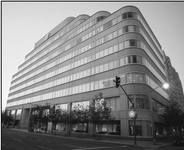
Administration Building 375 Eleventh Street, Oakland, 94607
