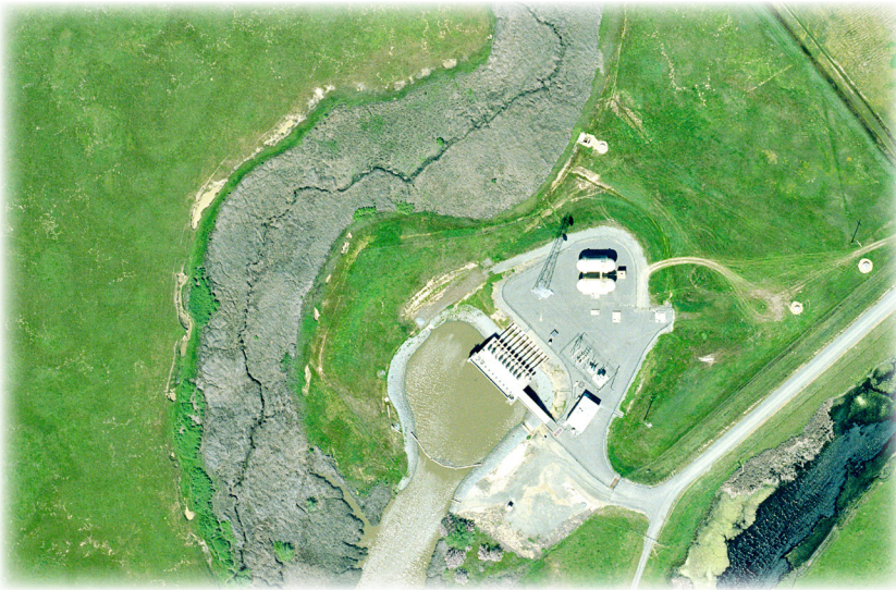
Barker Slough Pumping Plant
