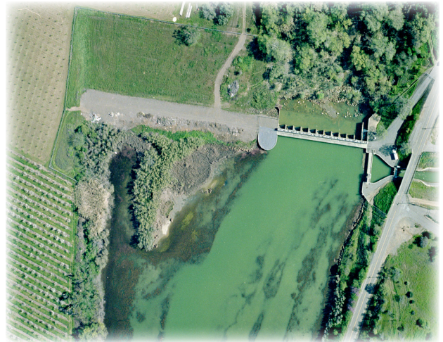
Putah Divison Dam
