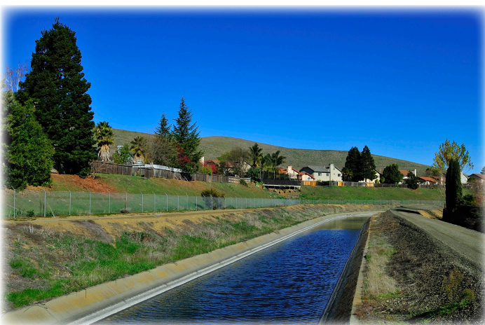
Putah South Canal
