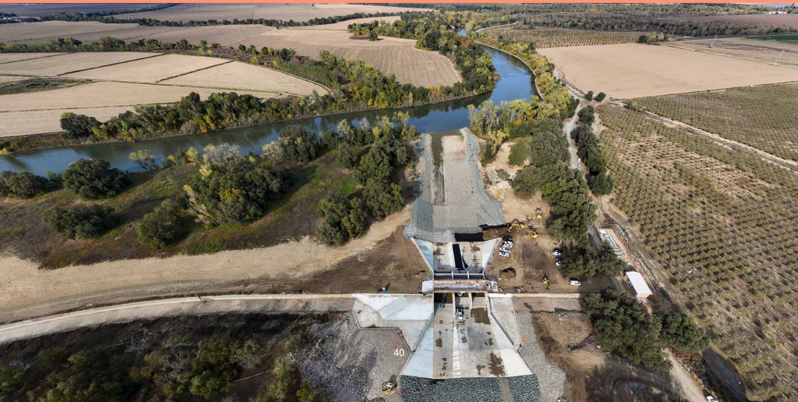
Drone view of Yolo Bypass Salmonid Habitat Restoration and Fish Passage (Big Notch) Project, courtesy CA Department of Water Resources.
