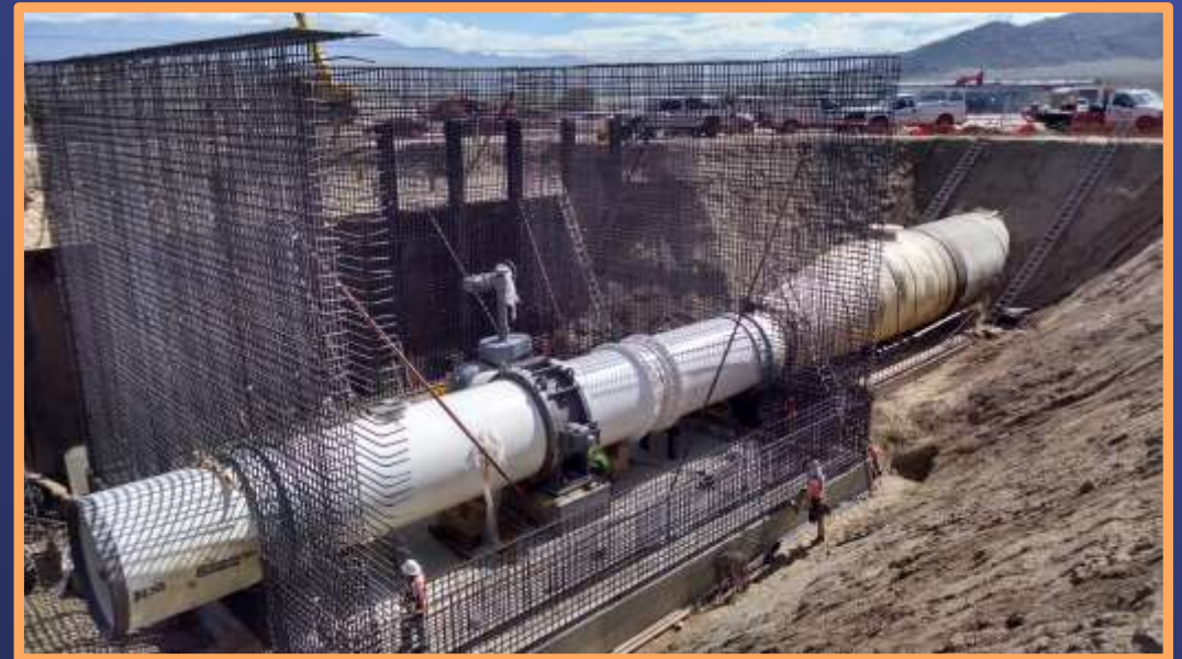
IF to Lakeview Vault Construction
