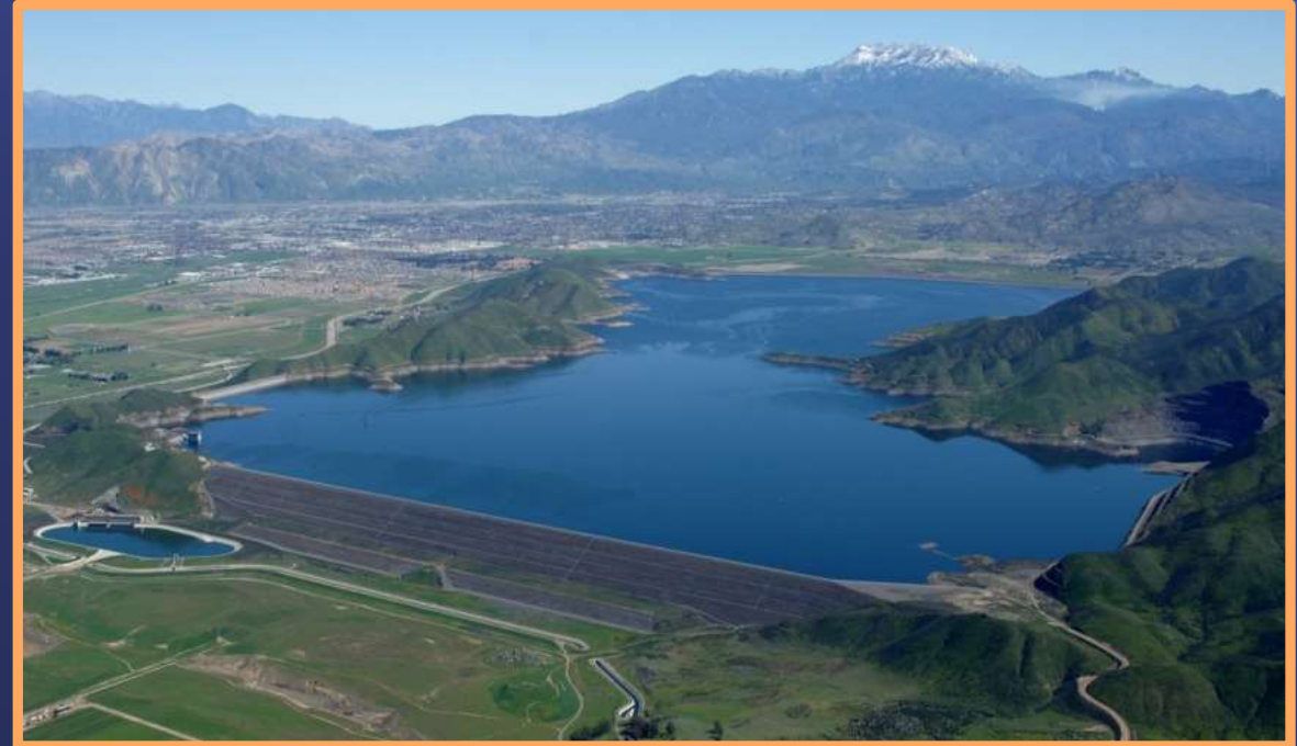
Diamond Valley Lake West Dam & Forebay
