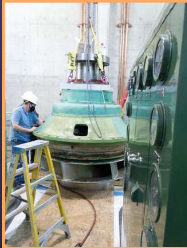
Iron Mountain – Impeller and Bearing Housing Removal
