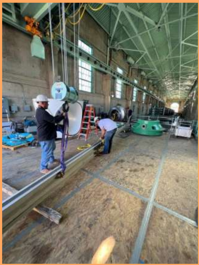
Iron Mountain – Crew using new crane during CRA pump and discharge valve rehab work
