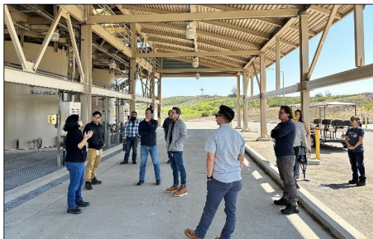
Plant engineers visiting the sulfuric acid tank farm at Skinner plant, spring 2024
