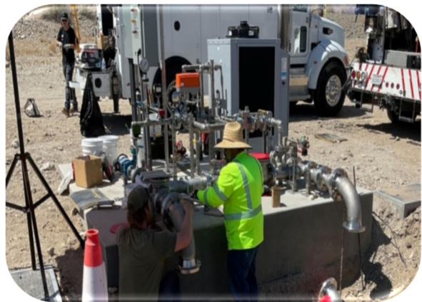
Eagle Mountain Domestic Water Chiller
