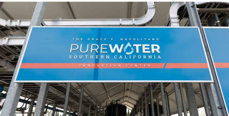
Pure Water Southern California demonstration facility
