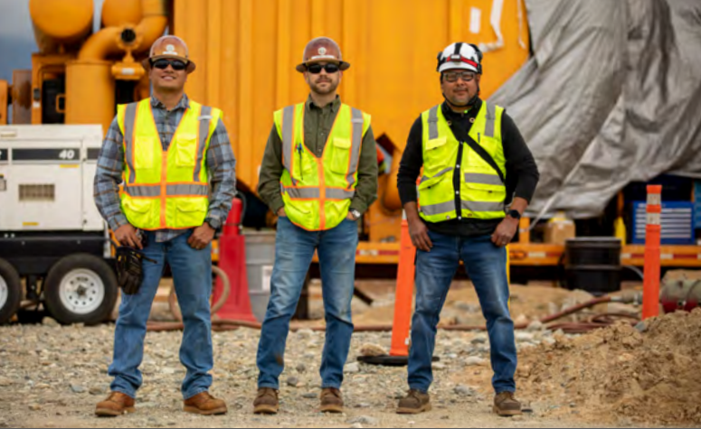
Starting the day at the Etiwanda Pipeline Re-liner during Phase 3.
