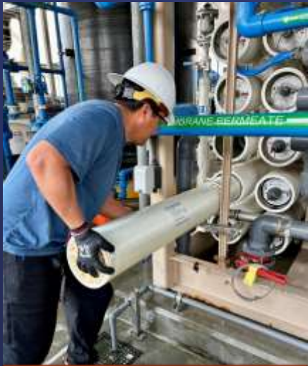
RO Element Installation
