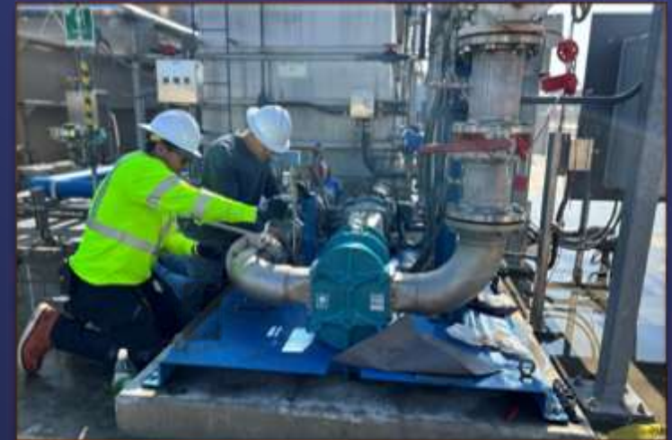
MBR Filtrate Pump Replacement
