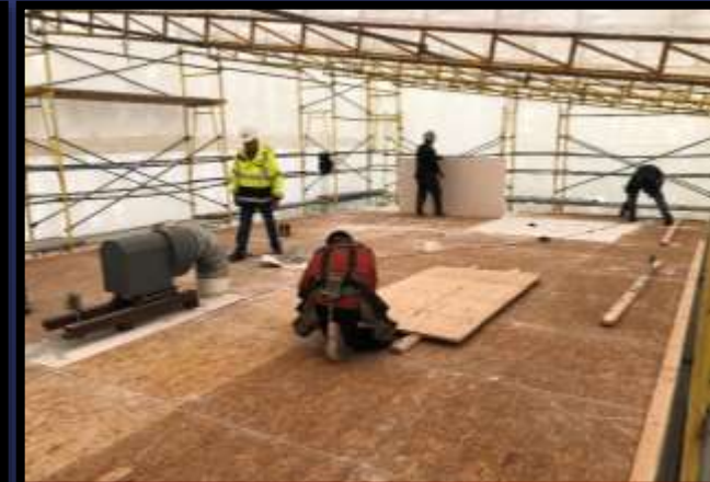
Operations Trailer Roof Replacement
